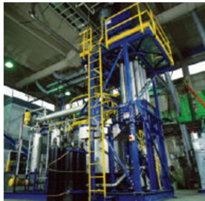
Pilot Plant at Canada 15 tn /day
