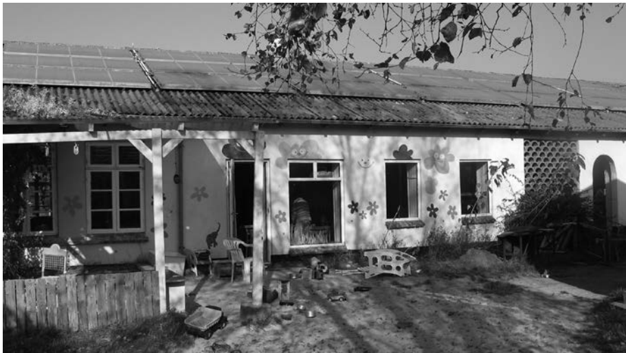
Figure 2: View of Toustrup Mark's kindergarten.
