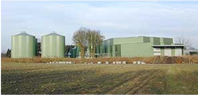
AD/CHP Plant in Germany, 8.4 MW
