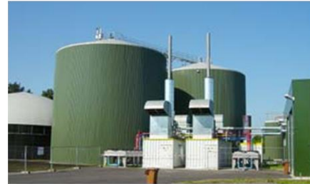
AD Reactors 2 X 3.000 m 3 , AD/CHP Plant 2.6 MW Germany
